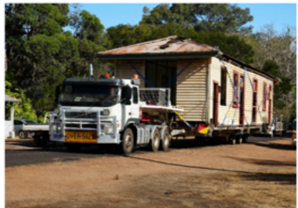
Relocating the North Greenbushes Railway Station
