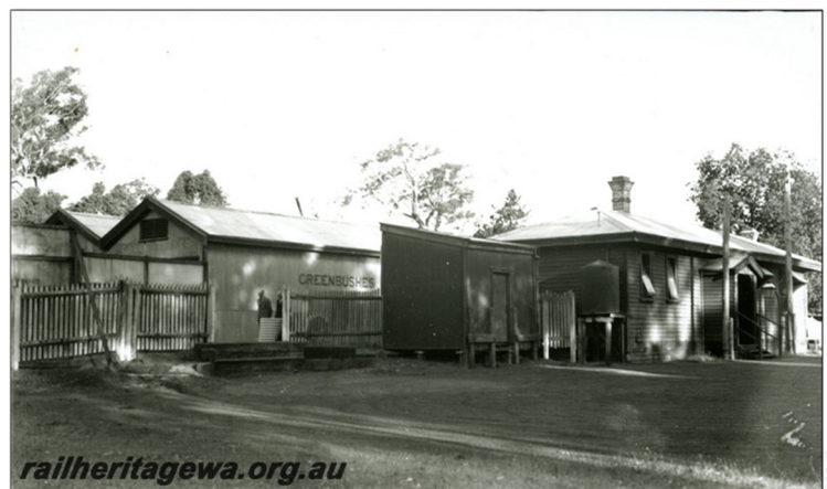
P22938 Station buildings, sheds, Greenbushes, PP line, view from road
